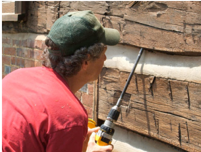
Sampling from the exterior of the Sheller Cabin in Smithville, Ohio
